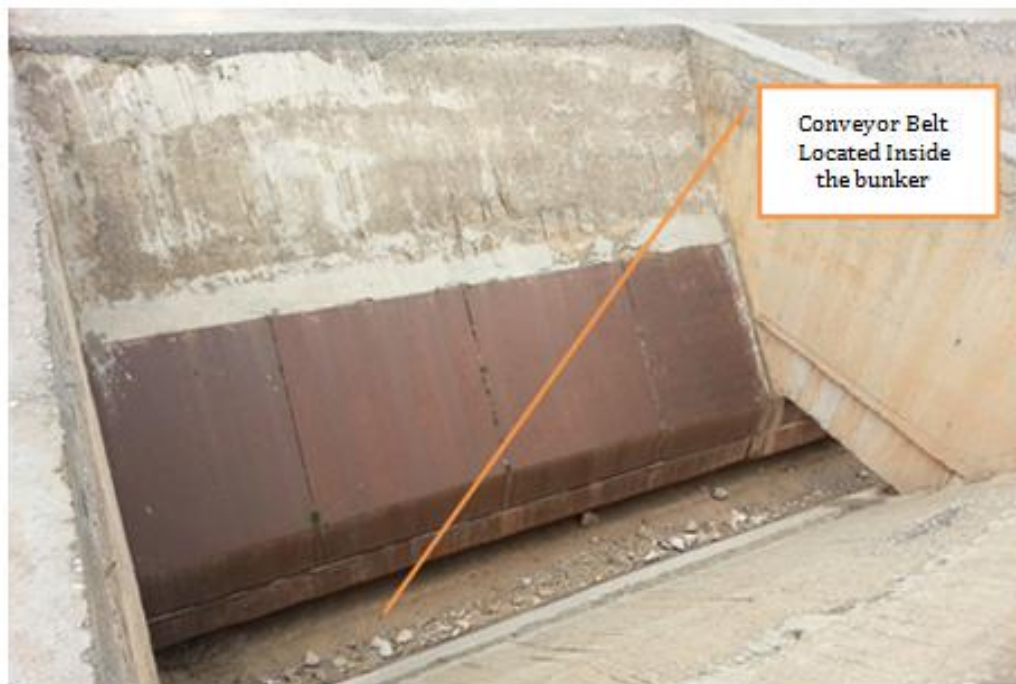
Figure 9 Conveyor Belt 1 Which is Located Inside the Bunker
