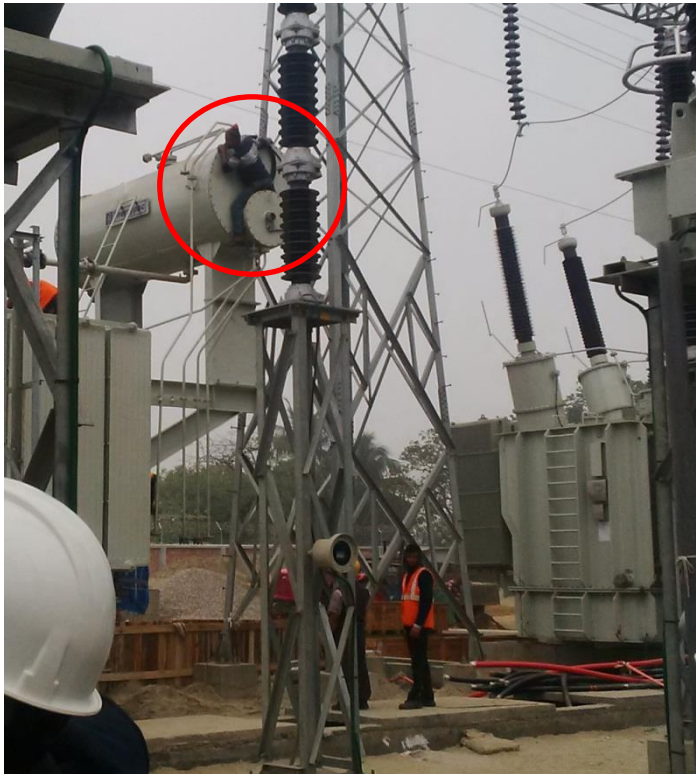
Figure 3.5: Labourer working at height in switchyard - no PPE, no safety harness, no working platform
