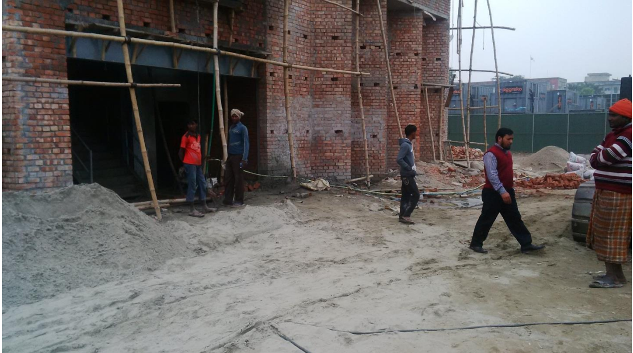
Figure 3.3: Construction workforce – no PPE (hard hats, high visibility jackets, safety shoes)
