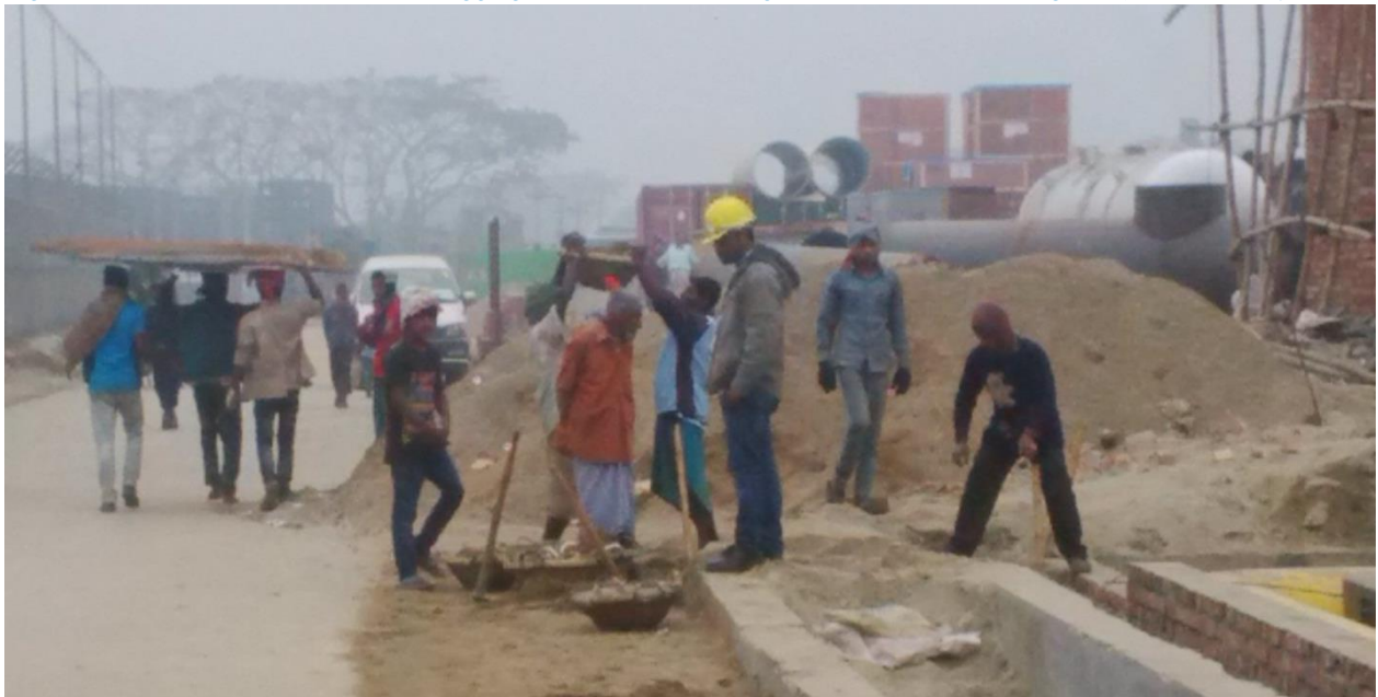
Figure 3.4: Construction workforce digging and manual handling - no PPE (hard hats, high vis jackets, safety shoes)
